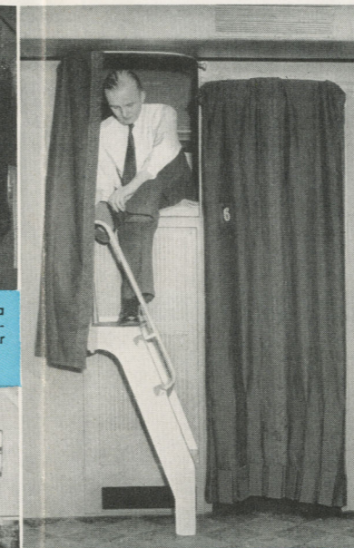
Protruding curtains greatly facilitate dressing in upper as well as lower berths in the new Pullman sleeping cars. Individual steps for upper berths automatically fold up when not in use and are entirely removed in the daytime or when space is used as a section for single occupancy.
