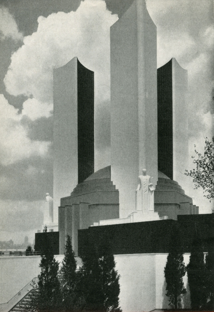
The magnificent Federal Building
