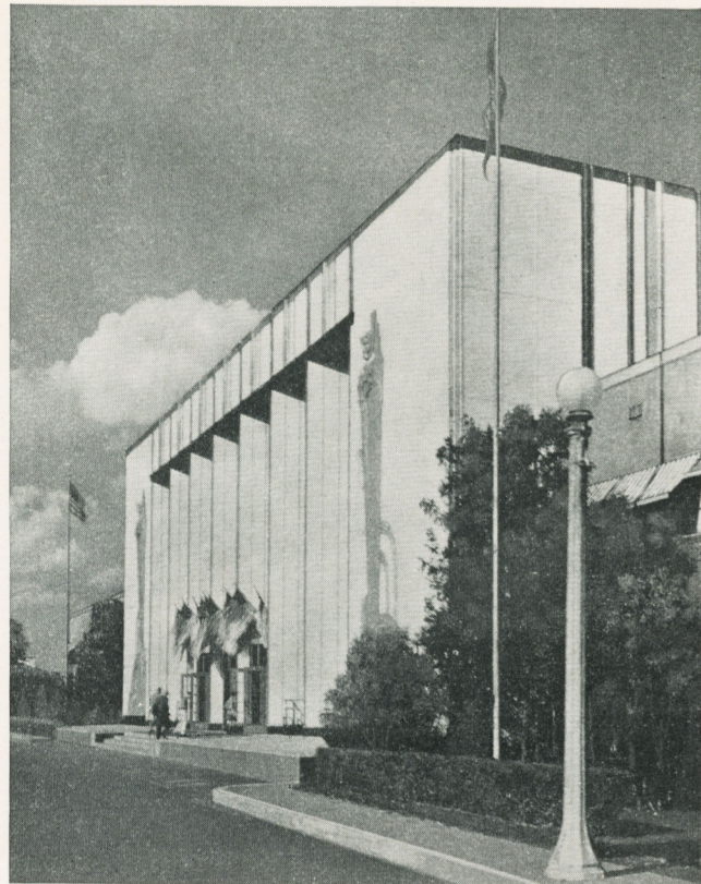
Administration Building, executive headquarters of the Exposition.
