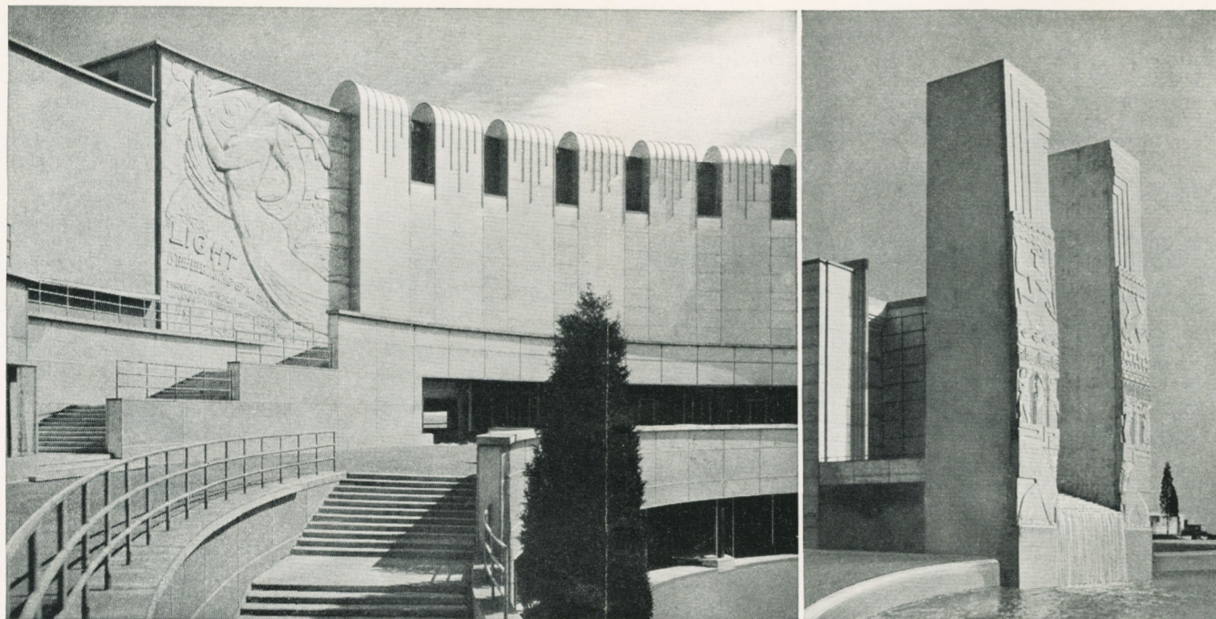
The beauties of architectural treatment are exemplified by the Electrical Building and its "Water Gate."
