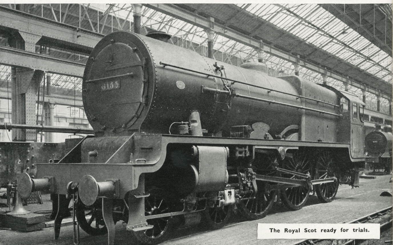
Boiler clothed, Cab in position and Locomotive being wheeled.
