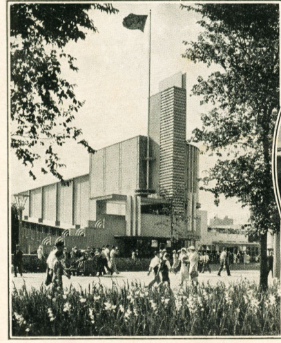
General Exhibits Building
