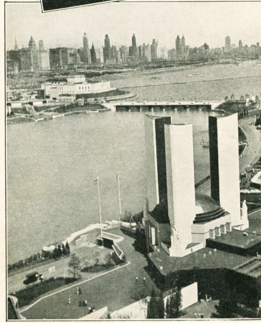
Federal Building and Chicago Skyline
