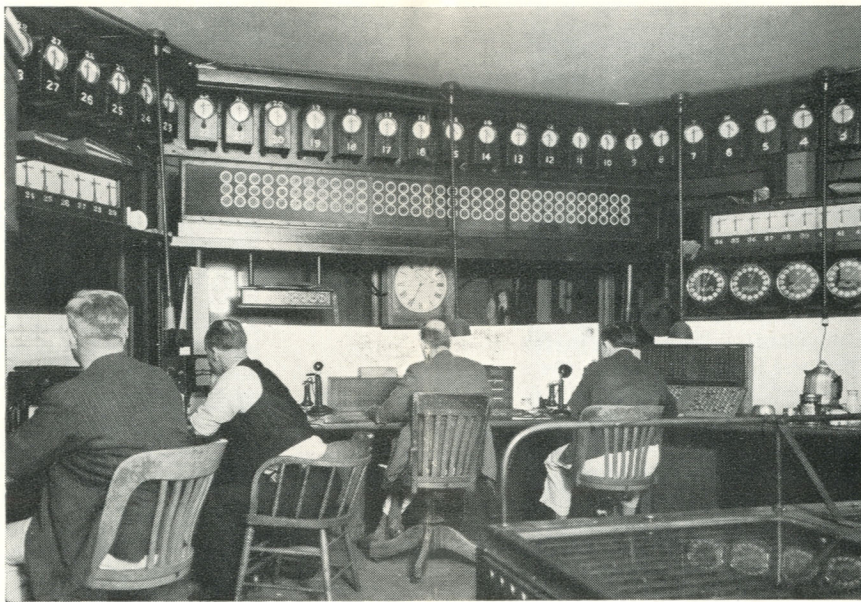
The operators in the Dispatcher's Office at Tower K, Washington Terminal, giving orders to the levermen who operate the switches and signals, all interlocked
