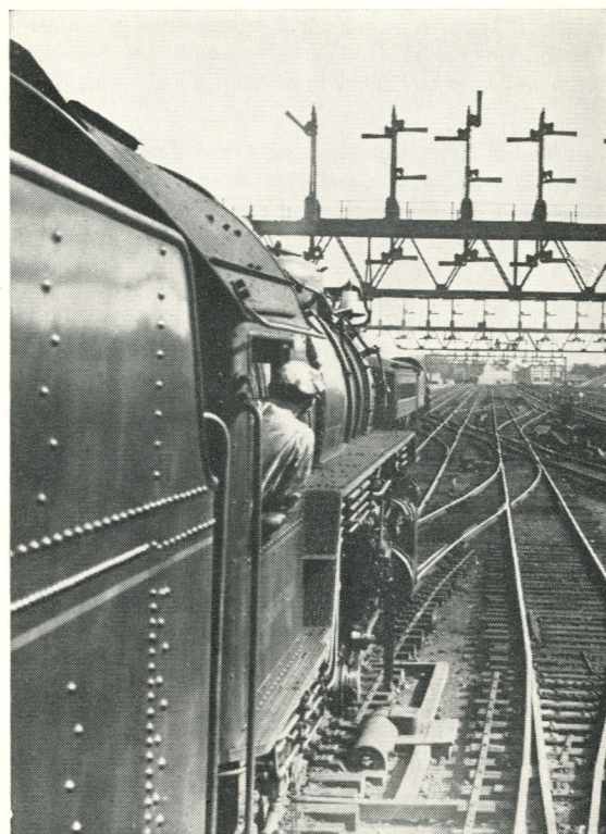
The engineer protected by interlocking systems gets his orders to leave the Washington Terminal
